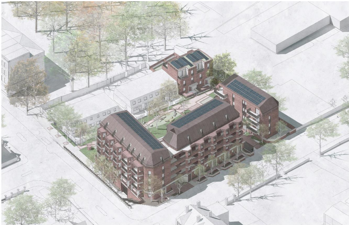
Figure 7: Cranwood House Scheme which includes erection of three buildings providing 41 homes which has been designed to Passivhaus standards, with very high fabric efficiencies and air tightness, triple glazed windows, a communal air source heat pump system, and solar photovoltaic panels on the roofs.
