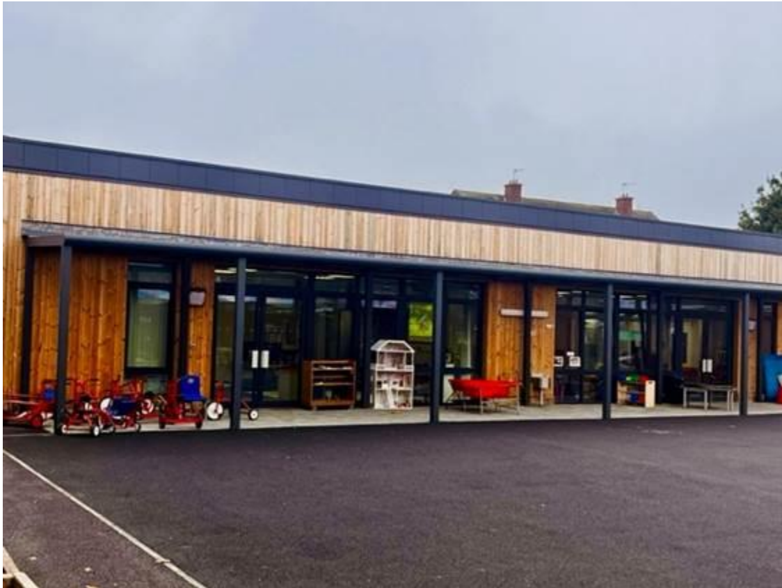
Figure 8: The new nursery building at Lordship Lane Primary School has two classrooms and is equipped with an air-source heat pump and photovoltaic panels which is a zero-carbon scheme.
